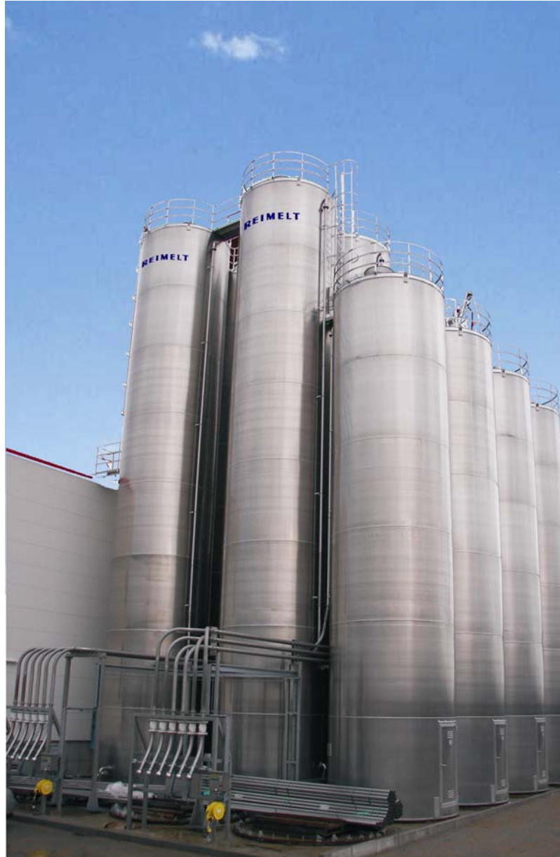
Picture 1: Outdoor silos for storage of raw material
